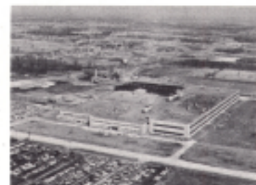
The Livonia Manufacturing Plant
