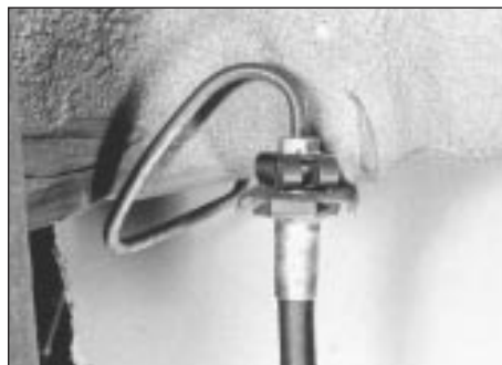
11.2 Rigid pipe-to-flexible hose connection
